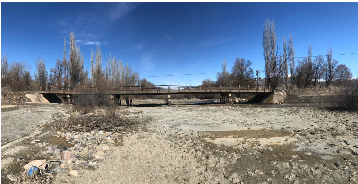
Fig. 4. Photograph of the bridge.
