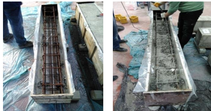
Fig. 2. Preparation of molds for concrete beams (Karalar 2020).
