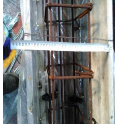
Fig. 2. Preparation of molds for concrete beams (Karalar 2020).
