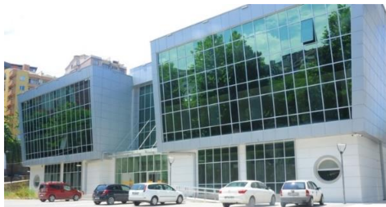
Fig. 9. General view of library building.
