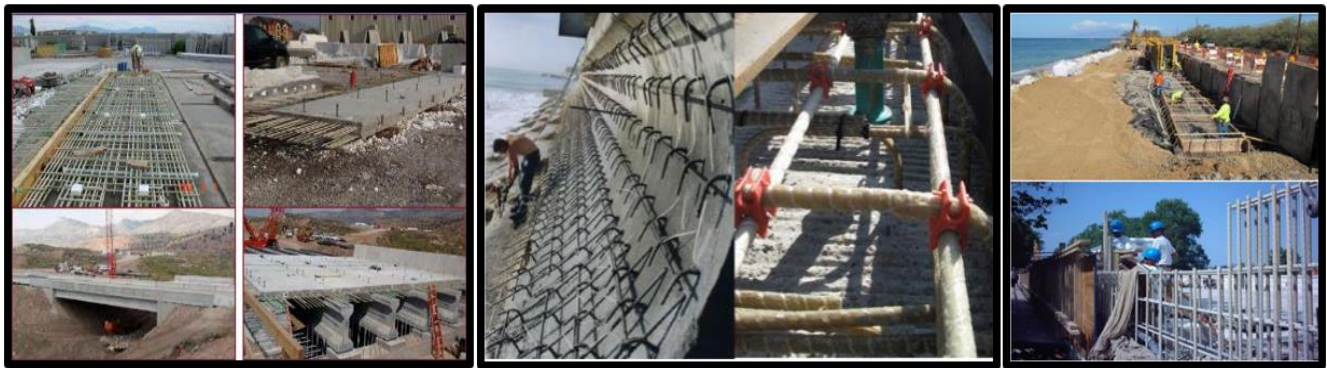
Fig. 1. Application areas where GFRP is used.
