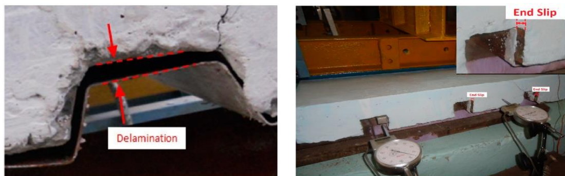
Fig. 2. Delamination and end slip in profiled sheet deck slab (Avudaiappan et al. 2021).
