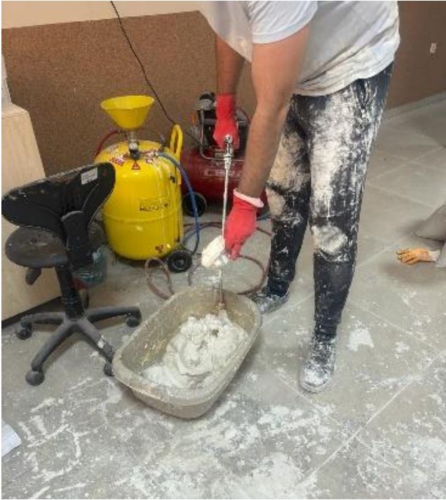
Fig. 2. Foamed concrete production.
