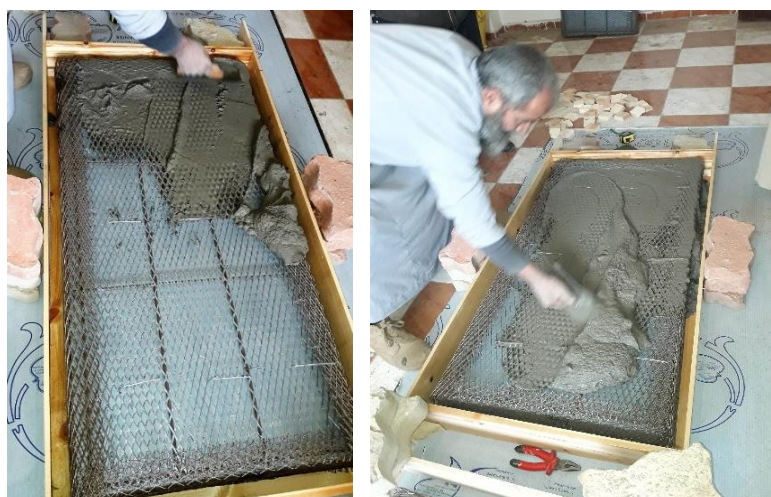
Fig. 7. Casting of concrete mix.
