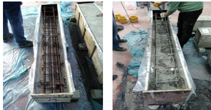
Fig. 2. Preparation of molds for concrete beams (Karalar 2020).
