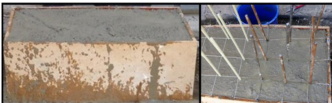
Fig. 3. Concrete production and rebar placement.
