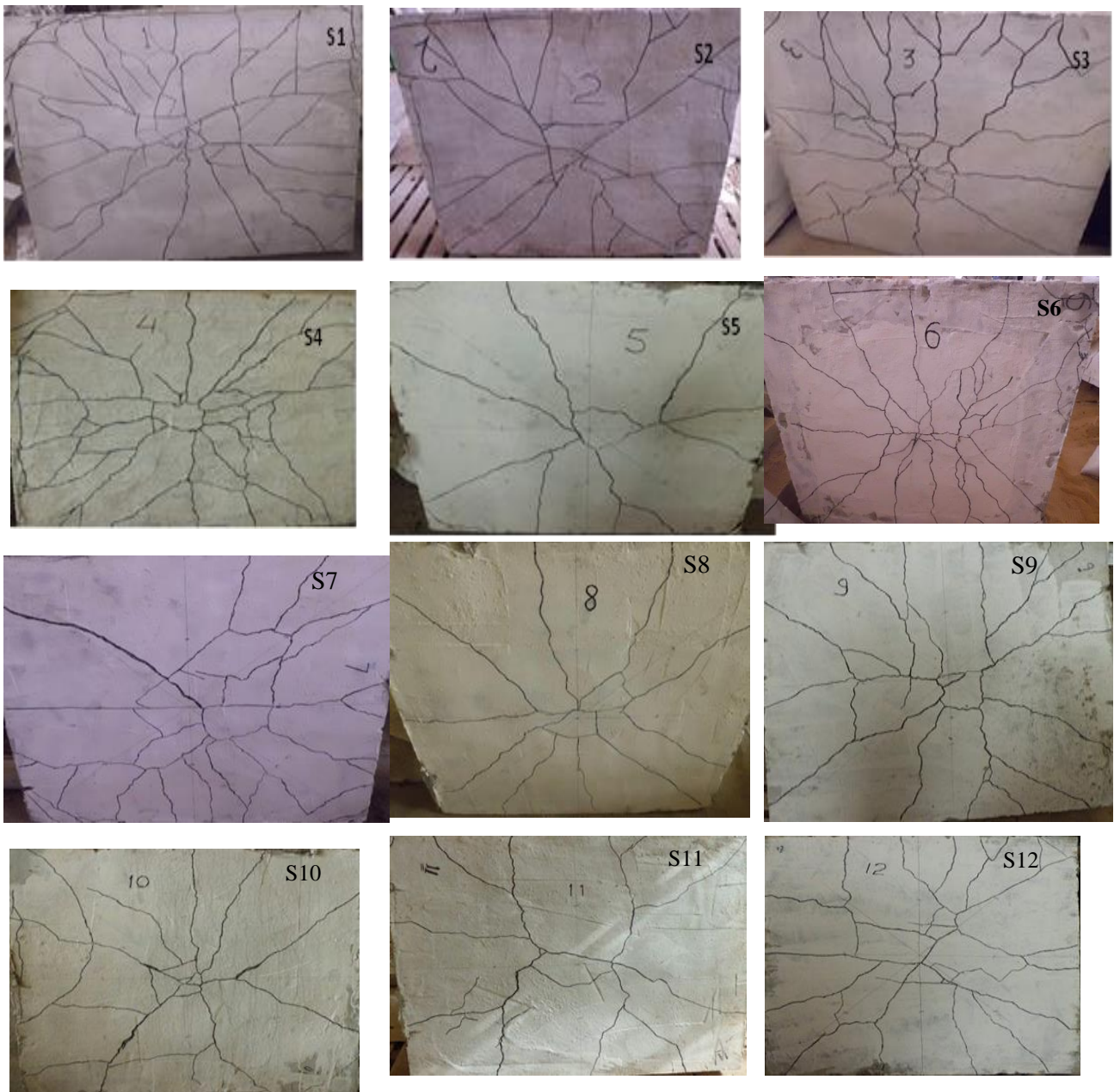
Figure 9: Cracking Pattern of Tested Slabs.
