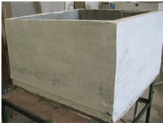
Figure 3. Healthy Ferrocement Tank.
