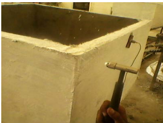
Figure 5. Experimental Test for the Tested Tank.
